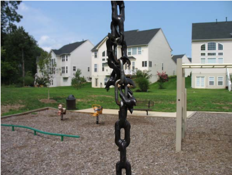
Photo 13 – Damaged swing chain behind 8724 Lords View Lp.
